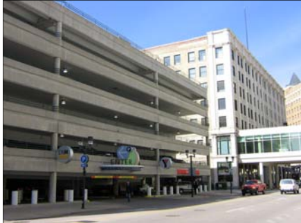
Attached parking structure
